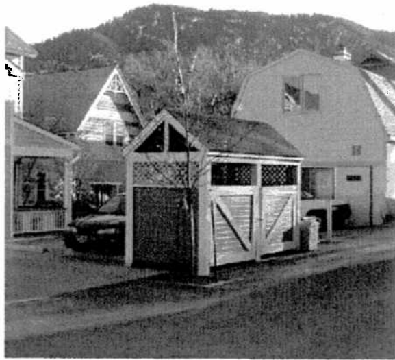
Figure 14-41. A well-designed service enclosure designed compatible with the multi-family buildings.
