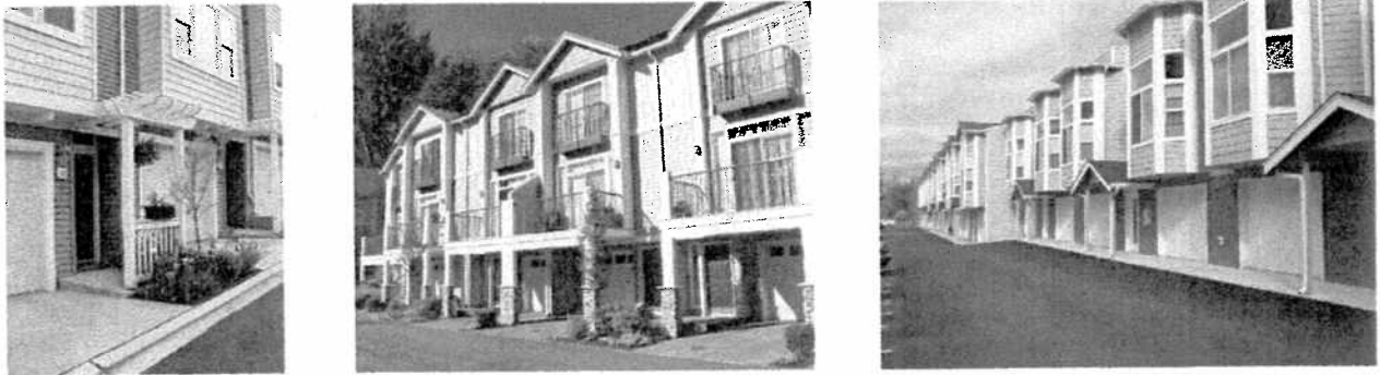
Figure 14-22. Good and bad examples of garage/entry configurations. The left example features a landscaped area and a trellis to highlight the entry. In the middle image, the balconies and landscaped areas de-emphasize the garage. In the right image, the lack of landscaping is a glaring omission.
