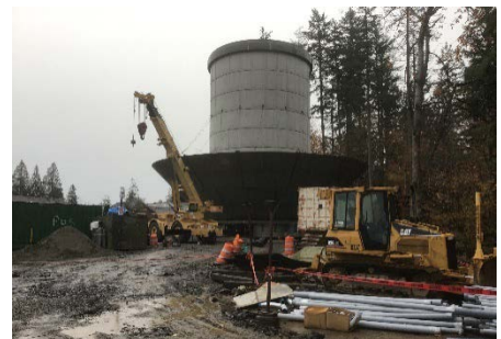
Constructing the Terry Cargil Reservoir
