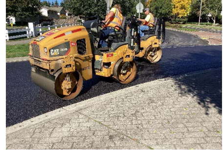
Compacting/rolling the newly laid asphalt in the roundabout at Rainier Rd and Balustrade Blvd in 2023
